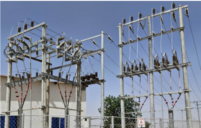
Interconnection point of the Zawaciki IMG, showing the incoming 33 kV line with its associated current transformer and energy meter.
